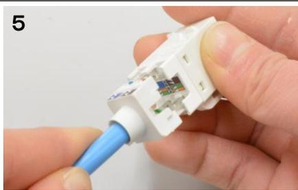
◆ Temporarily fix with reference to the wire cap and the mark of the main body.
