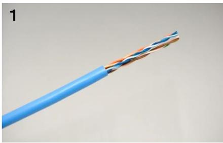
◆ Remove the cable jacket about 40mm.
