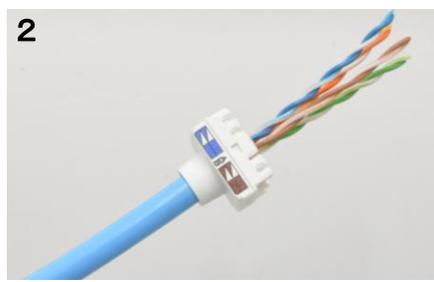
◆ Secure the cable to the wire cap.
